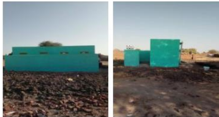
New constructed school sanitation facilities
